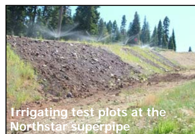
Constructing test plots at Heavenly
